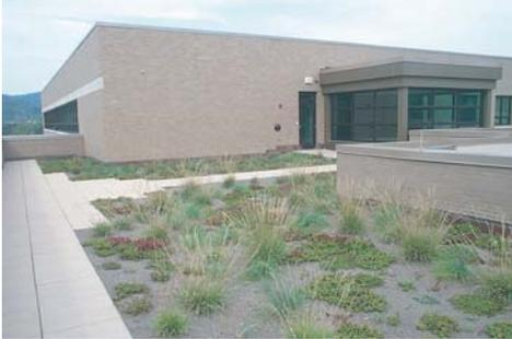
The District has installed a section of vegetated roof over its main office building. This roof consists of a six-inch soil medium, planted with decorative grasses and other drought resistant plants. The purpose of this technology is to minimize the amount of runoff that occurs from rain falling on a rooftop. The soil and vegetation serve as a natural sponge that absorbs smaller rain events without allowing any runoff.
