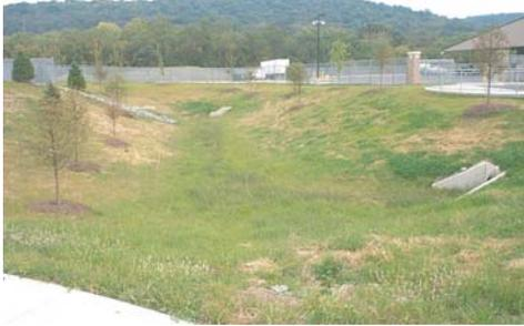
A dry detention basin is dry until a storm event occurs. Depending on the intensity and duration of the storm, the basin is designed to control the peak rate of storm water runoff from the site to a level that does not exceed pre-development conditions.
