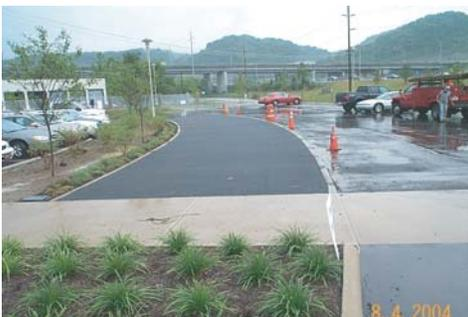
Unlike conventional asphalt pavement, permeable asphalt is a porous pavement that allows water to drain through it. This pavement can be designed to handle traffic loadings and has been successfully used in many parts of the country, particularly in parking lot applications. Permeable asphalt pavements achieve their porous characteristics by removing the fine aggregates from the mix design.
