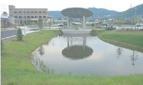
A retention pond is a constructed pond that maintains a permanent pool of water. Pollutant removal comes primarily by way of sedimentation. Solids, metals, nutrients in particulate form and organics are the target pollutants. Removal efficiencies are dependent upon the amount of time that runoff remains in the pond.
