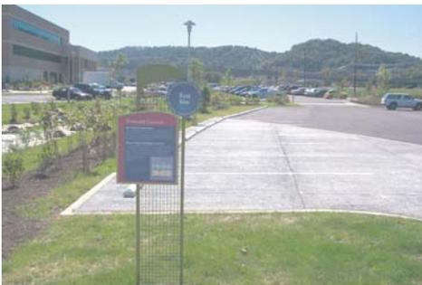
Permeable concrete pavement is another form of porous material that allows water to pass through it. This system has been designed to handle traffic loadings. Porosity of this pavement is likewise achieved through selective use of aggregate material that creates void spaces between the larger stone material.
